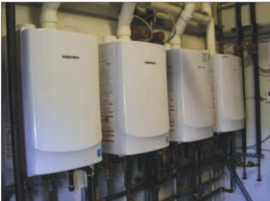
Navien condensing water heaters have one of the highest gas efficiency ratings on the market, with up to a 0.96 rating.
